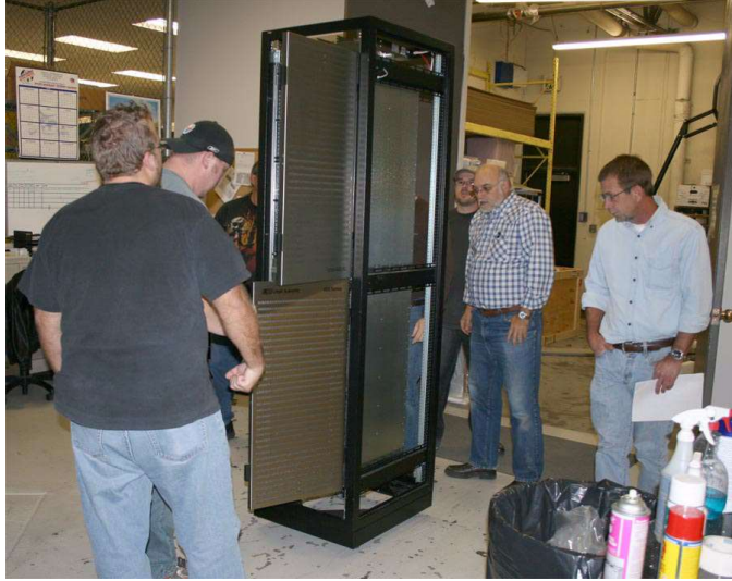
FIGURE 2-14. Rack upright, ready for final location move
