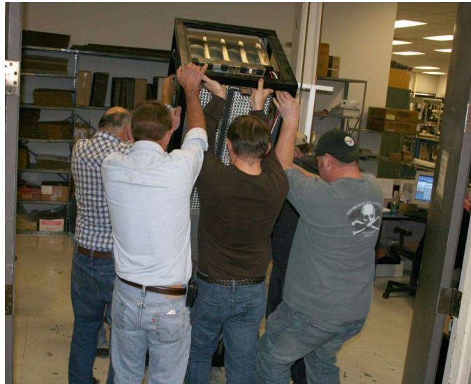
FIGURE 2-13. Rack brought upright
