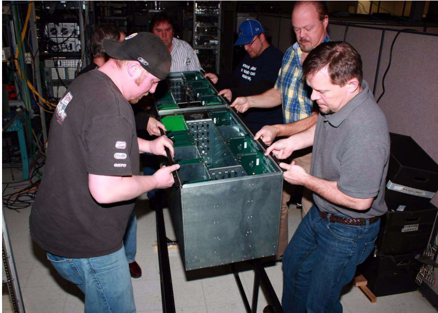
FIGURE 2-17. XL chassis lift and carry
