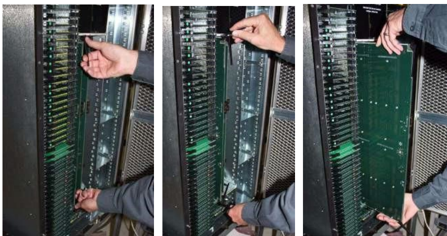
Crosspoint Board Removal
